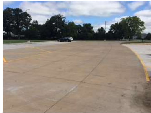
Parking Lot Modification
