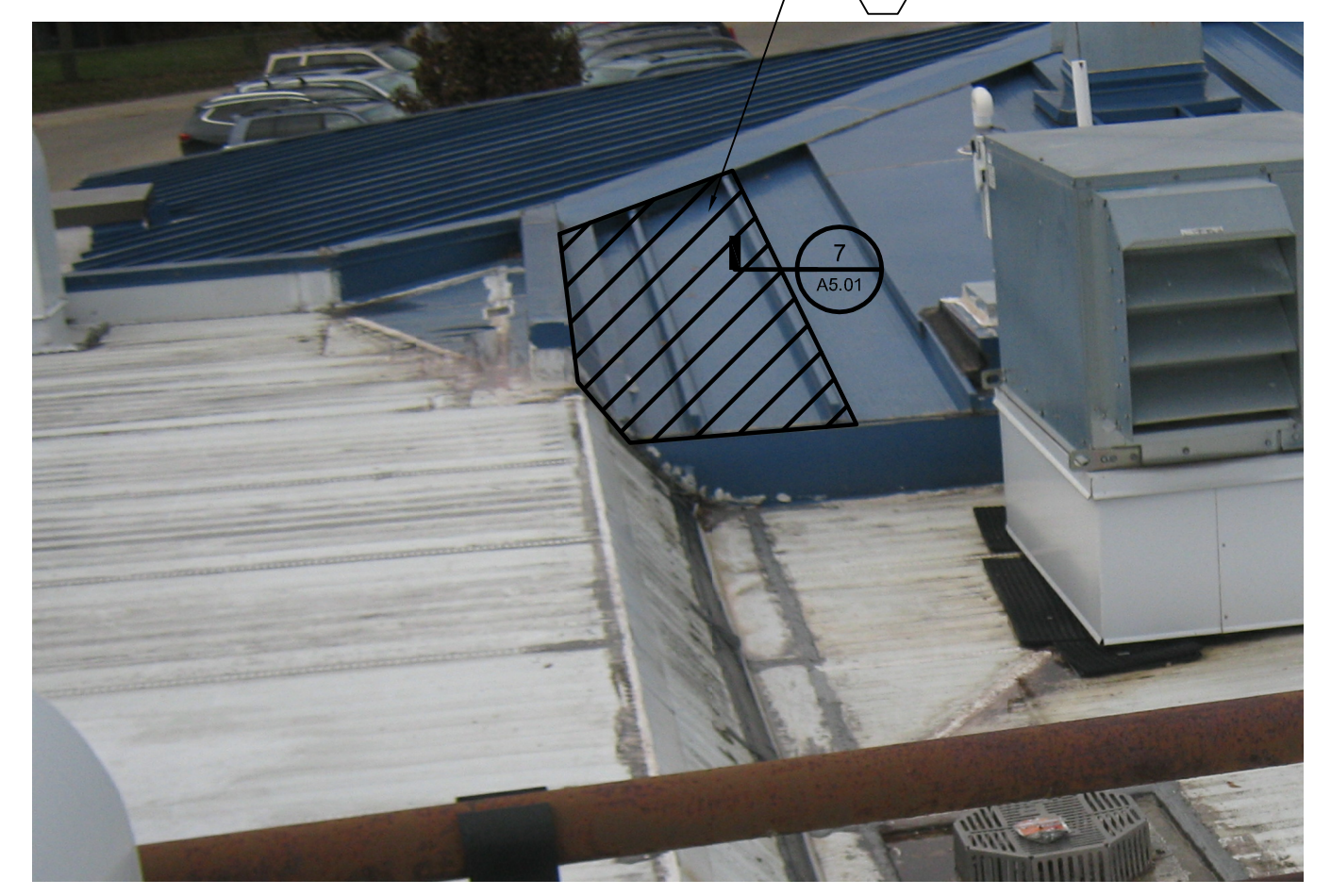
5 REFERENCE PHOTO - ROOF FLASHING NOT TO SCALE
