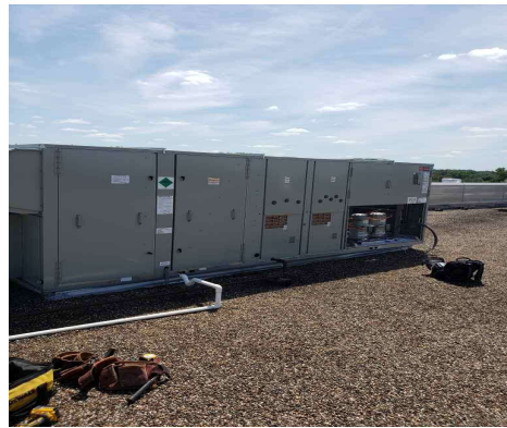
NEW HVAC UNIT
