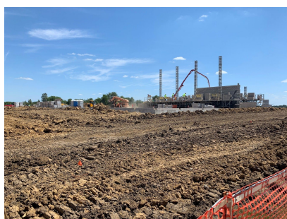
First walls at Hazel Point
