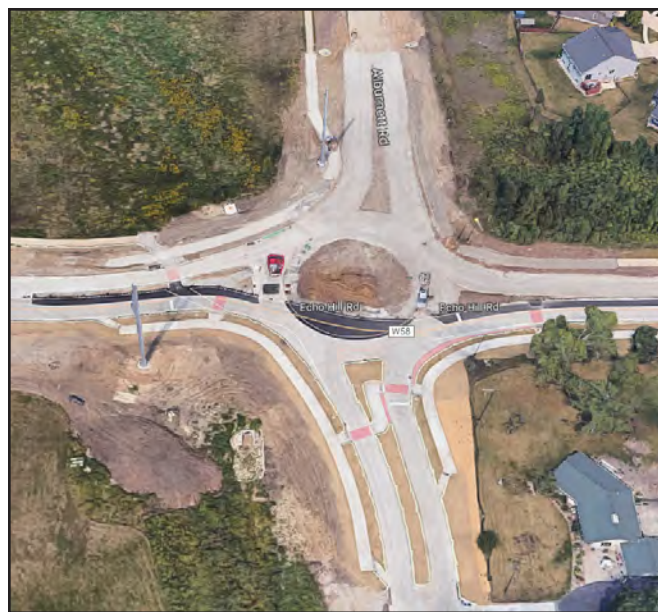
Construction of the roundabout at Echo Hill Road and Alburnett Road. It opened in the fall of 2022.
