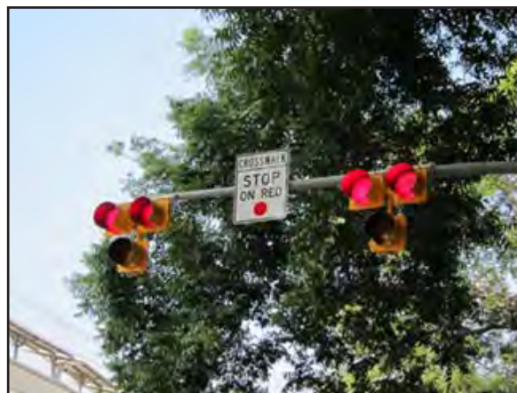
Image 35: Example of a pedestrian hybrid beacon on a stop light arm mast. Source: Federal Highway Administration
