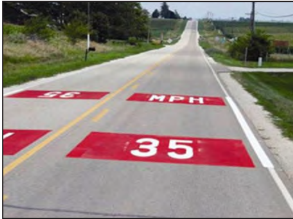
Example of Speed Limit Pavement Legend with Red Background Source: Federal Highway Administration
