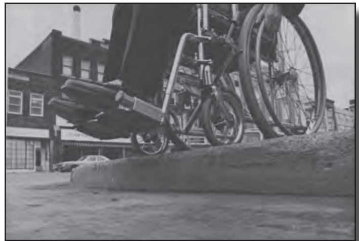
Figure 48: An inaccessible curb. Curb cuts were installed after World War 2 for veterans with disabilities and physical limitations.
