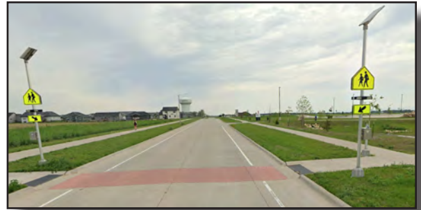
Figure 51: The RRFB on 35th Street in front of Boulder Peak Intermediate. While it may be tempting to stop to let a child out here instead of pulling into the school site, it adds to hazards on the streets - for all roadway users.
